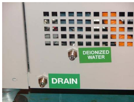
DI Water Input and Drain Ports (Left View)
